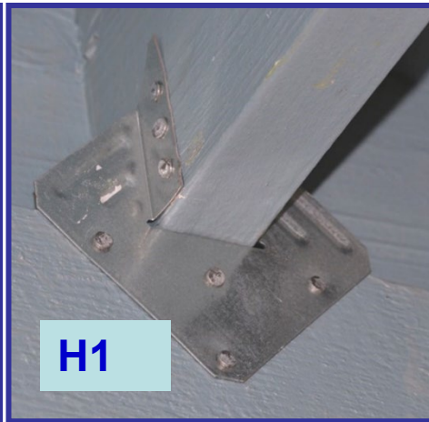
H1 Clips - Roof to Wall Tie - Stronger than Code.
